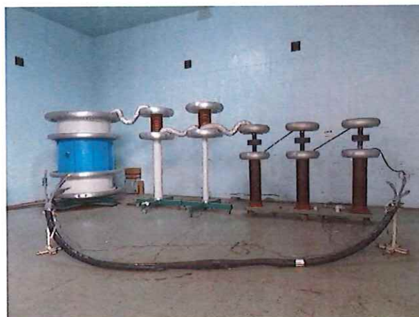
G2: 样品局部放电试验及交流耐压试验 Partial discharge test and AC voltage test on the sample
